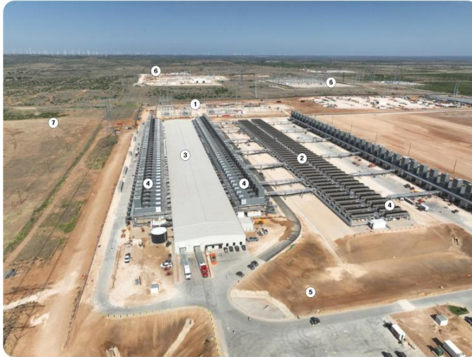
Phase I of the Helios Data Center campus, July 2026.
