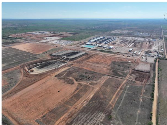
Galaxy's Helios Data Center campus, April 2026.
