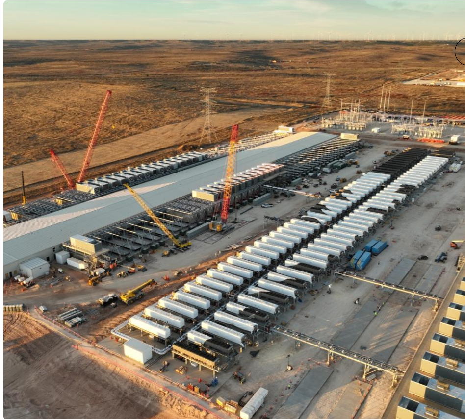
Galaxy's Helios Data Center campus under construction for Phase I, January 2026.
