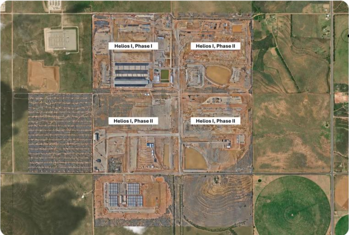
Aerial view of a portion of the Helios campus, featuring Helios I, Phases I and II, under development as of October 2026. Image does not depict the full 2,200+ acres under Galaxy's control; capacity figures are campus-wide unless otherwise noted.
