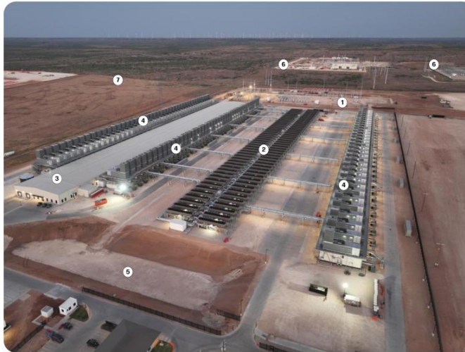
Phase I of the Helios Data Center campus, September 2026.
